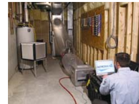
The Aeroseal technology injects aerosolized vinyl polymer particles into a pressurized duct system. The particles stay suspended in the air stream until they reach leaks, where they are deposited and build up at the leak edges until the leaks are sealed.
