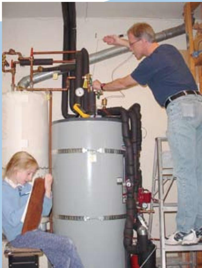
I know that my tank is 119 gallons (450 l), and I know that the shape of the storage area is roughly an upright cylinder. With a little math, I can chop up the water column into 1-foot (0.3 m) "slices," figure out the average temperature per slice, and calculate the Btu that this represents. If I take the temperature-versus-depth readings in the morning and again in the evening, I've got the daily Btu harvest and can now compare the "pump on" and "pump off" configurations, right?
