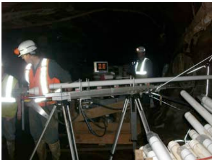
Figure 5: Golder crew-Wayne Mulder (middle) and Christopher Phillips (right)-of Mississauga, Ontario, Canada insert Televiewer column into drill hole
