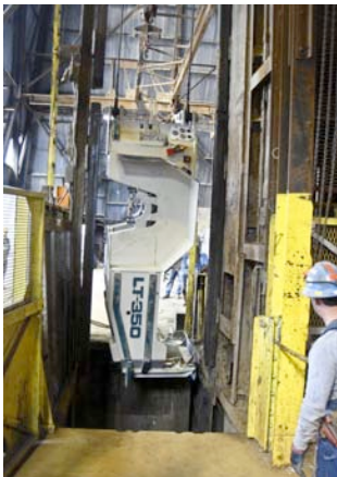
Figure 12: LHD arrives at 4850 Level below the Ross Shaft cage
