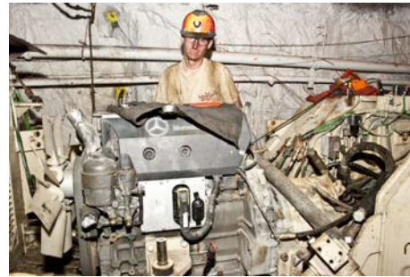
Figure 13: Josh Rouns of MTI assembles the LHD at the 4850 Level Crossover. Please note Mercedes engine logo.
