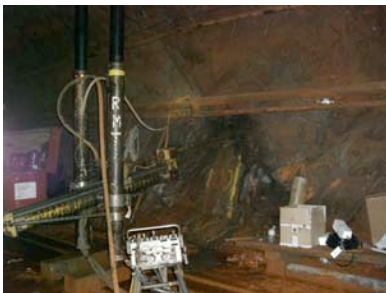
Figure 6: Drilling/overcoring of the instrument (Golder crew from UK)
