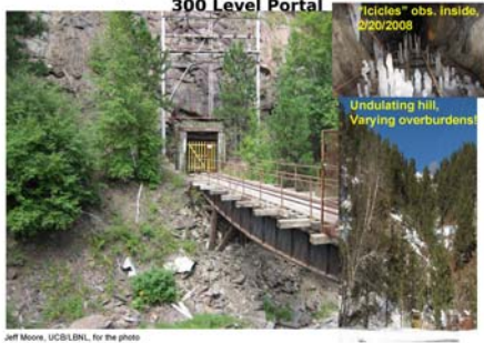
Frozen Seeps Observed along Oro Honto Drift with 300 Level Portal
