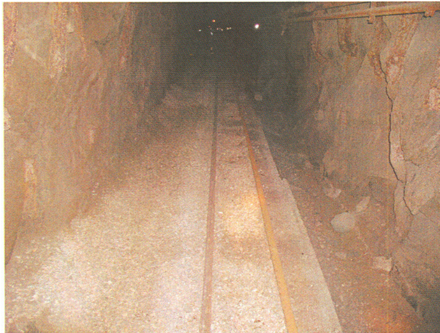
Photo 7. 2000 Level, 9 Ledge drift, limestone track ballast.
