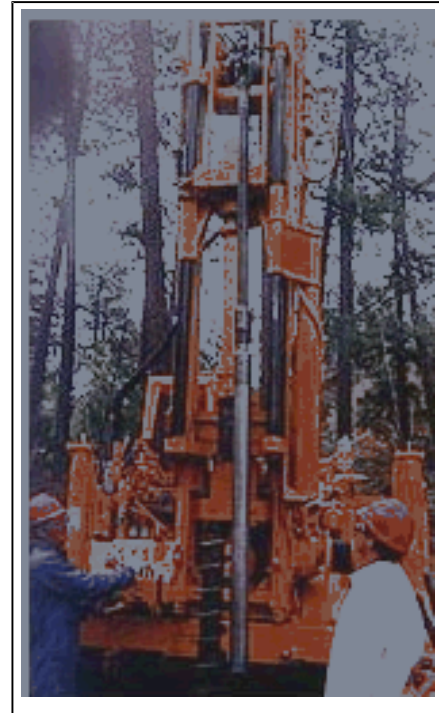
Figure A-1 Standard drill rig used for characterization activities
