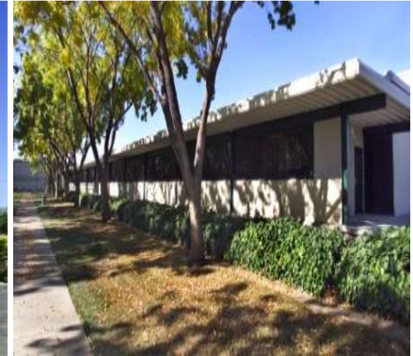
JOINT GENOME INSTITUTE Walnut Creek (~100,000 GSF)
