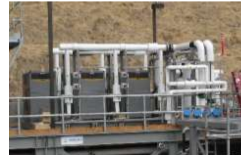
New efficient boilers
